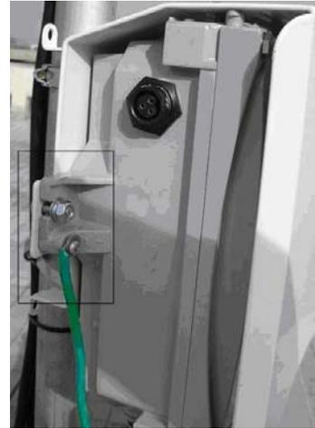
Figure 10. Grounding DWR-500.
